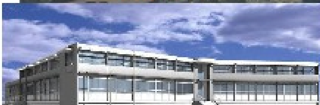
•Base Facility in La Serena
